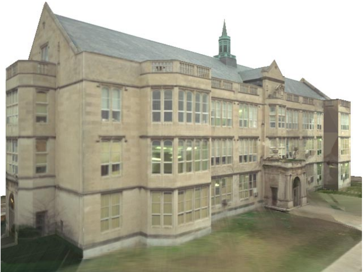
Figure 5.14: A synthetic view of University High School. This is a frame from an animation of flying around the entire building.
